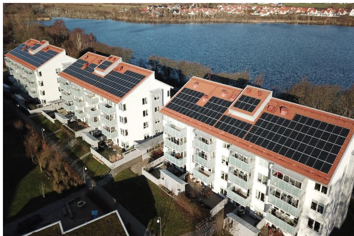
Figure 10. The BRF Kalkbrottet building complex.
